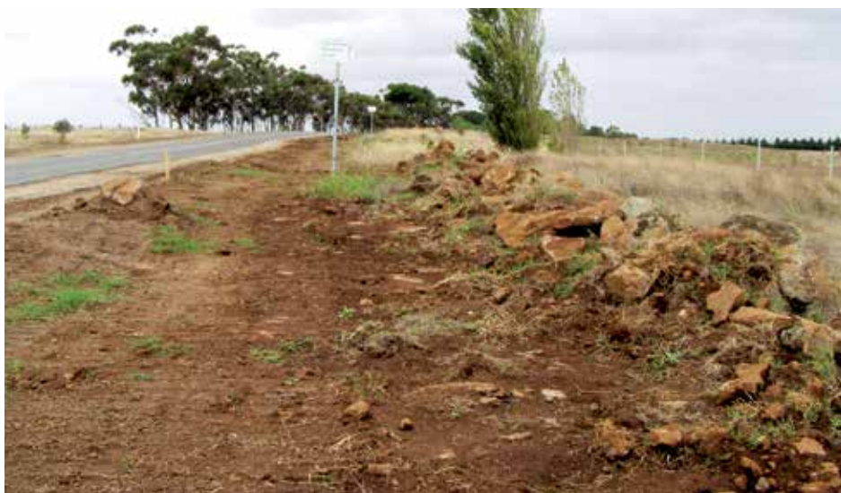
ABOVE: Roadworks impacting on a significant roadside
